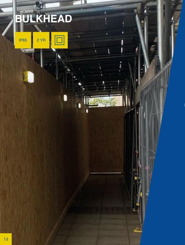
TAMCO's Bulkhead comes pre-wired with 500mm cable and includes a separate mounting bracket. It is a compact and durable solution for illuminating the work site, with an IP65 rating that makes it suitable for outdoor and indoor use. Featuring an impact resistant polycarbonate body, the bulkhead is a rugged wall light with multiple cable entries and an optional red diffuser.
